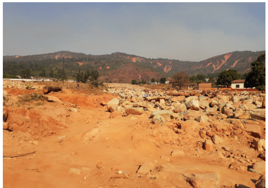
Trail of destruction, such is the impact of climate change. A picture taken from Chimanimani, Zimbabwe after cyclone Idai, showing the extent of damages caused by the cyclone in Zimbabwe, Mozambique and Malawi in 2019 - Photo: David Mukomana
