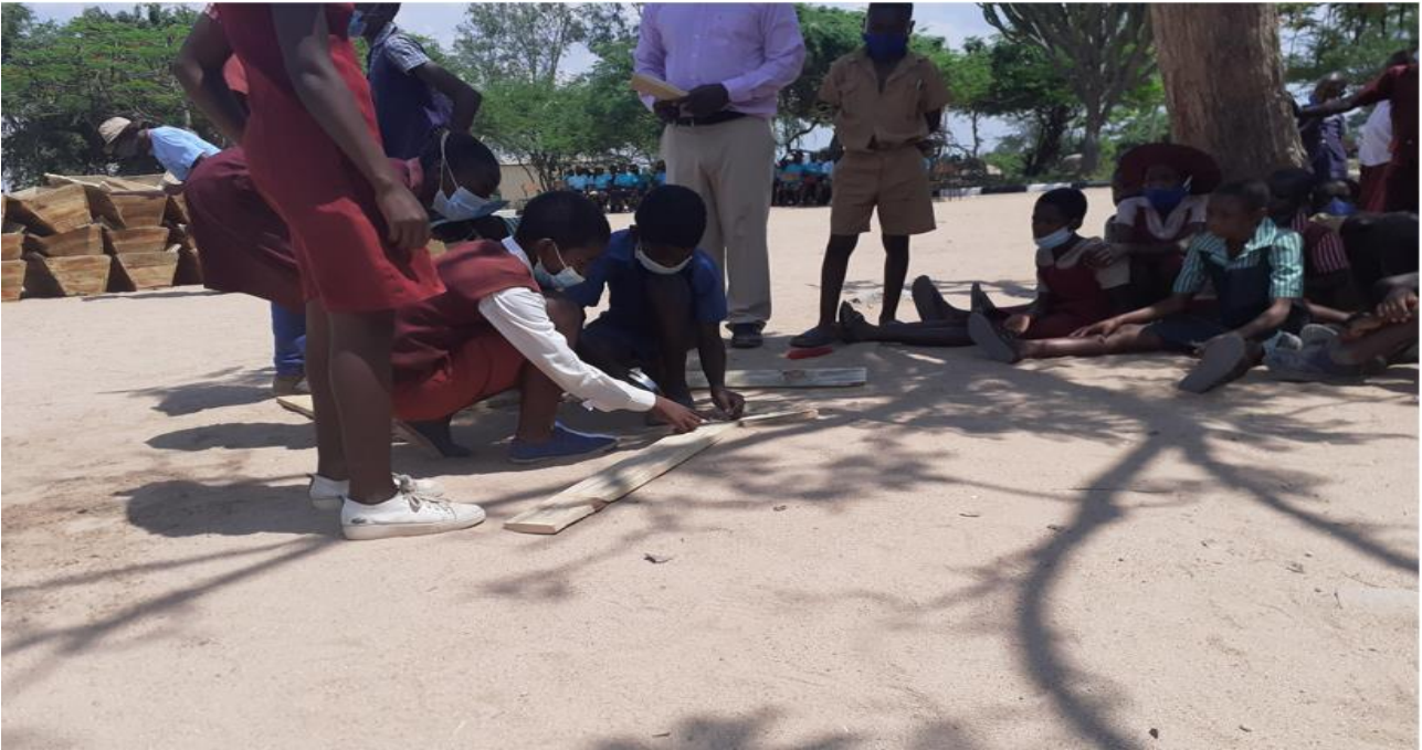
Picture above: The Primary Schools Team preparing their timber to start constructing the hive in front of the delegates.
